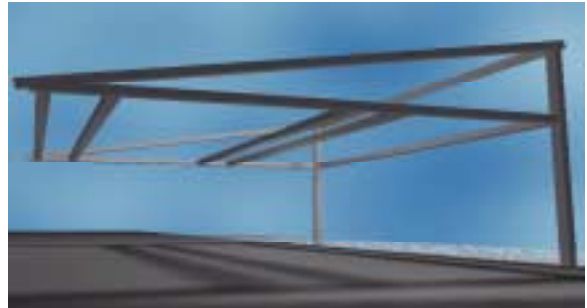
Fig. 2. View from the track side
